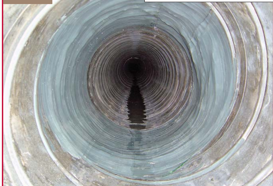
The cured liner gives the pipe a smooth, leak-free interior.
